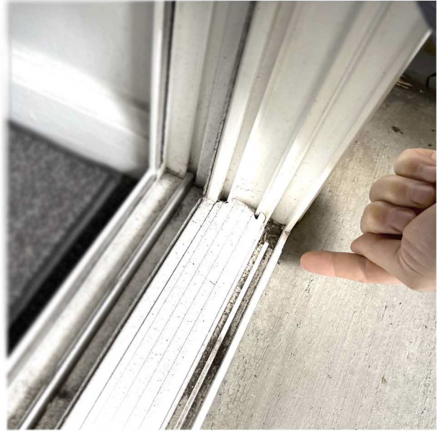
SLIDING GLASS DOOR TRACK - WEEP HOLE LOCATION
