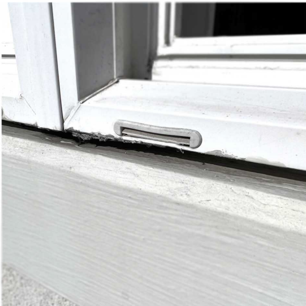
WINDOW - WEEP HOLE ON OUTSIDE
