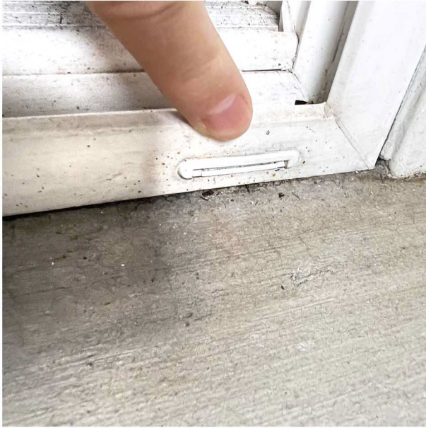
SLIDING GLASS DOOR TRACK - WEEP HOLE ON OUTSIDE
