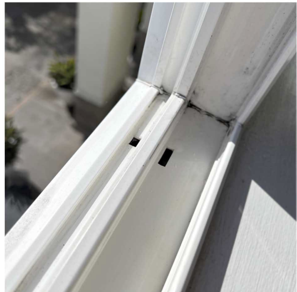
WINDOW TRACK DRAIN HOLES - THE WATER EXITS TO WEEP HOLES
