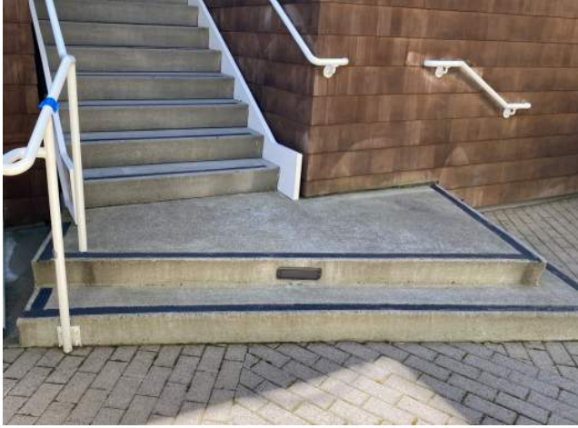
79: Stair by Unit 255
