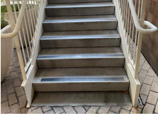
19: Stair by Elevator #3
