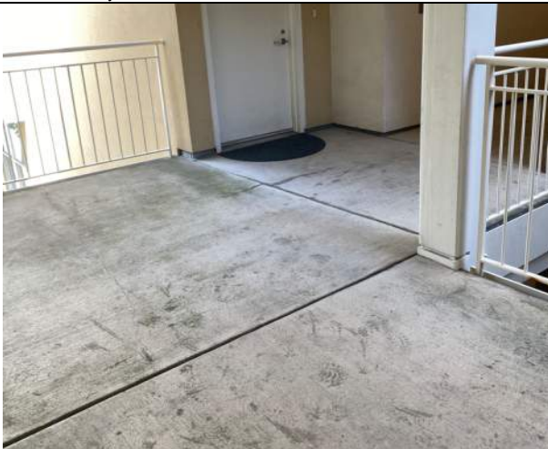
27: Stair by Elevator #3
