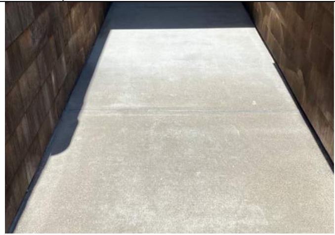
78: Stair by Unit 254
