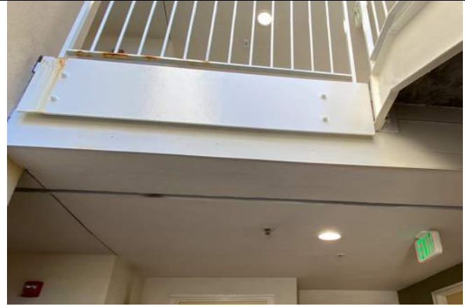
62: Stair by Unit 248
