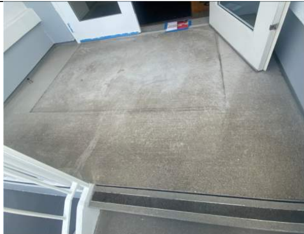
48: Stair by Unit 232
