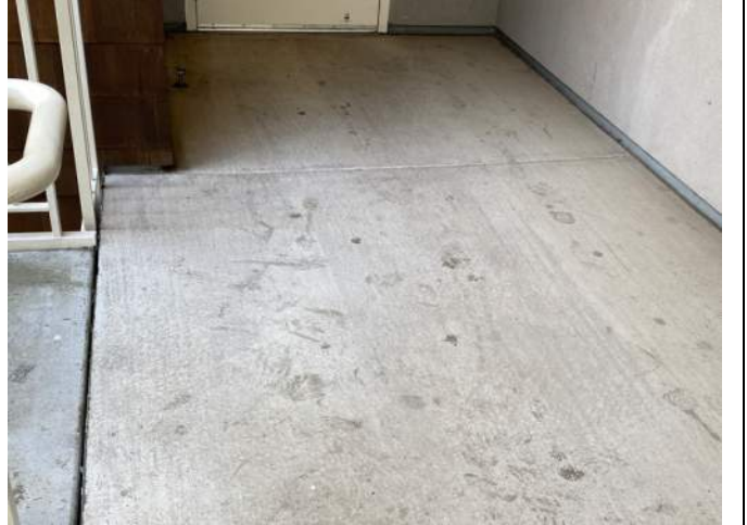
22: Stair by Elevator #3
