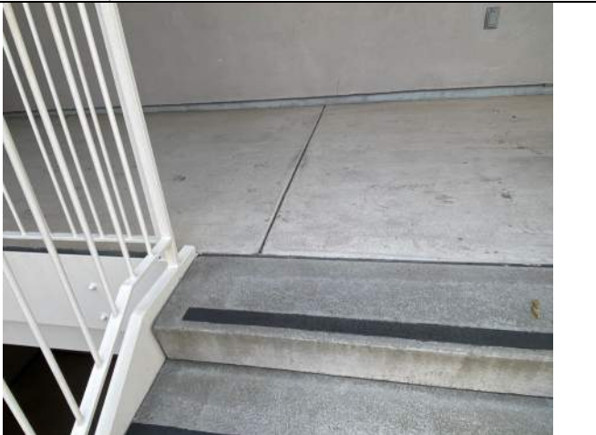
23: Stair by Elevator #3
