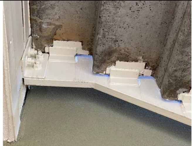
64: Stair by Unit 248
