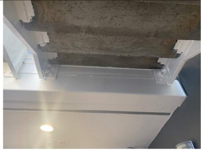
8: Stair by Unit 206
