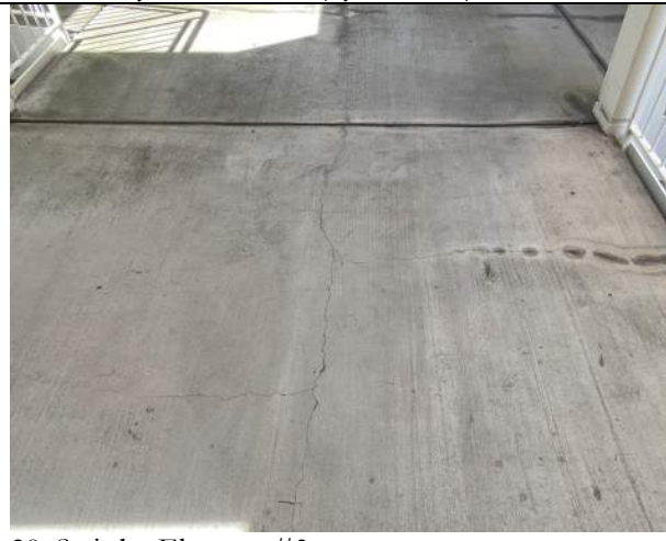
28: Stair by Elevator #3
