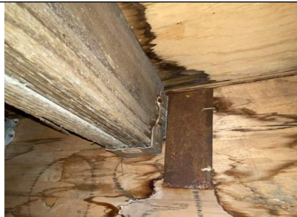
30: Stair by Elevator #3 (opened next to unit 216 from below)
