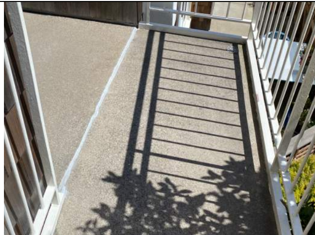
77: Stair by Unit 254
