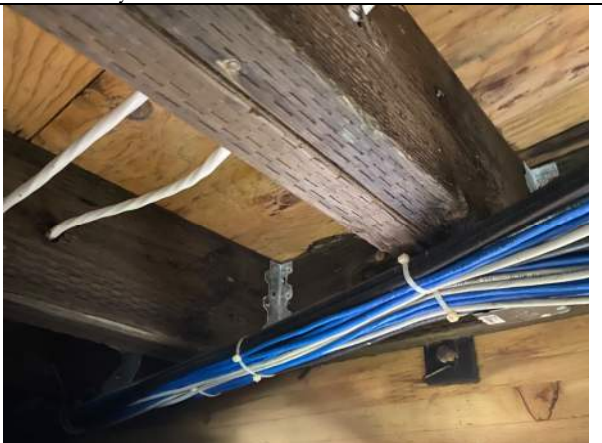
29: Stair by Elevator #3 (opened next to unit 218 from below)
