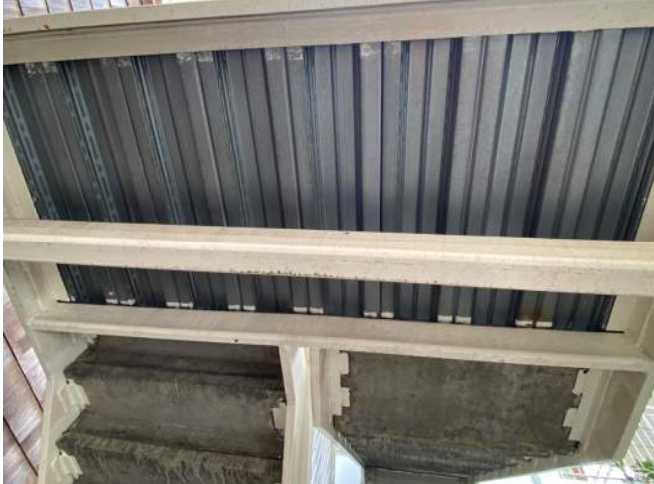
21: Stair by Elevator #3
