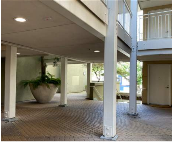
25: Stair by Elevator #3
