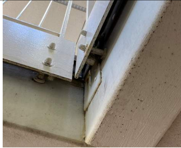
26: Stair by Elevator #3 (by unit 216)
