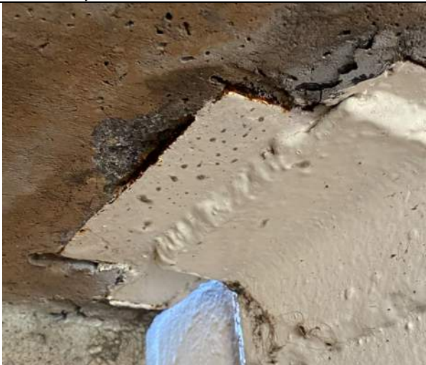
71: Stair by Unit 250
