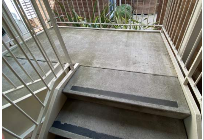
20: Stair by Elevator #3
